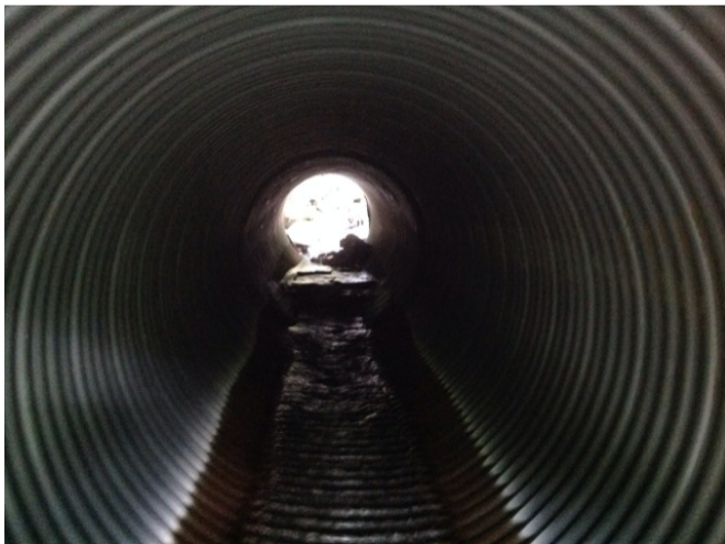
looking through culvert
